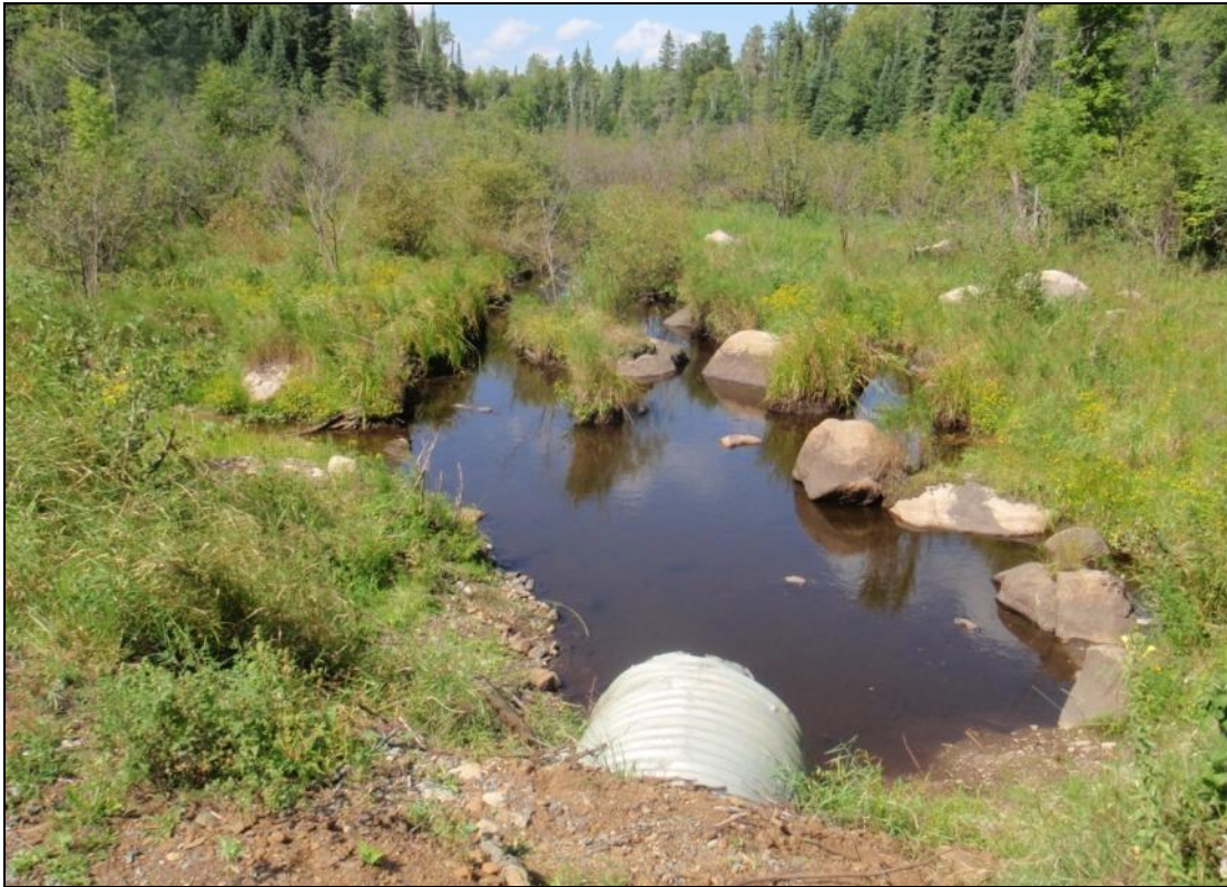
Looking upstream from culvert, August 2010.
