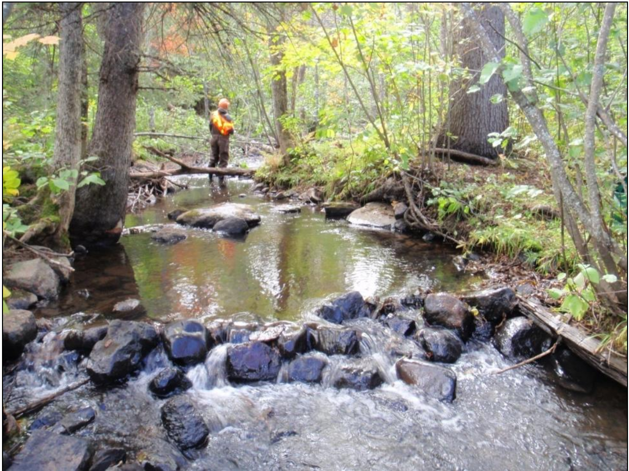
Figure 34. Rock dam at Site 16 on Whitewood Creek.
