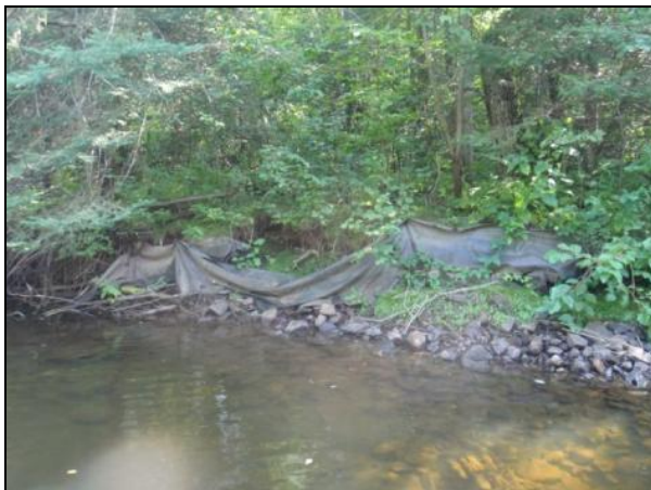
Figure 37. Geotextile used at Site 8 (L) and Site 9 (R; red arrow) to prevent erosion.
