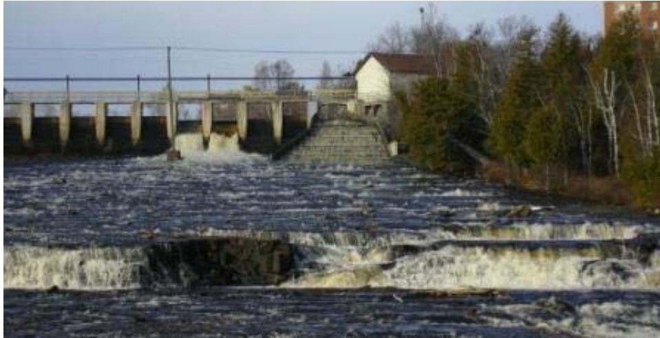
Current River Fish Ladder
