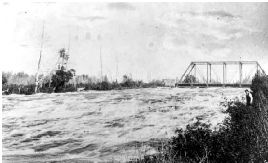
Original configuration of the CP Rail bridge, looking upstream from the mouth of the Current River.
