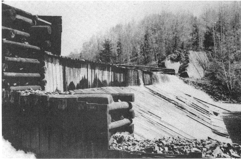
Onion Lake Dam, 1953 configuration. Upper timber section of the dam, looking east. — James F. Maclaren Ltd. 1970.
