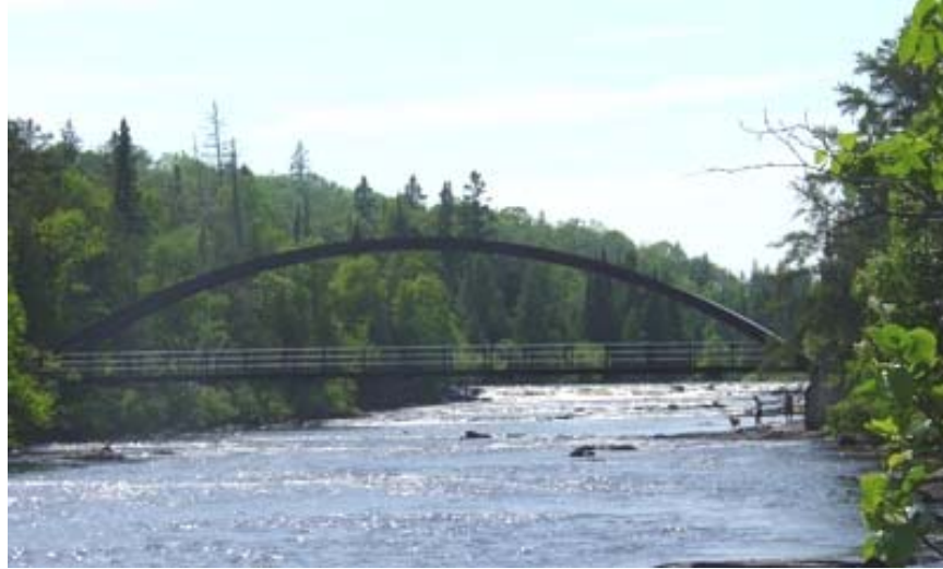
Trowbridge Falls pedestrian bridge
