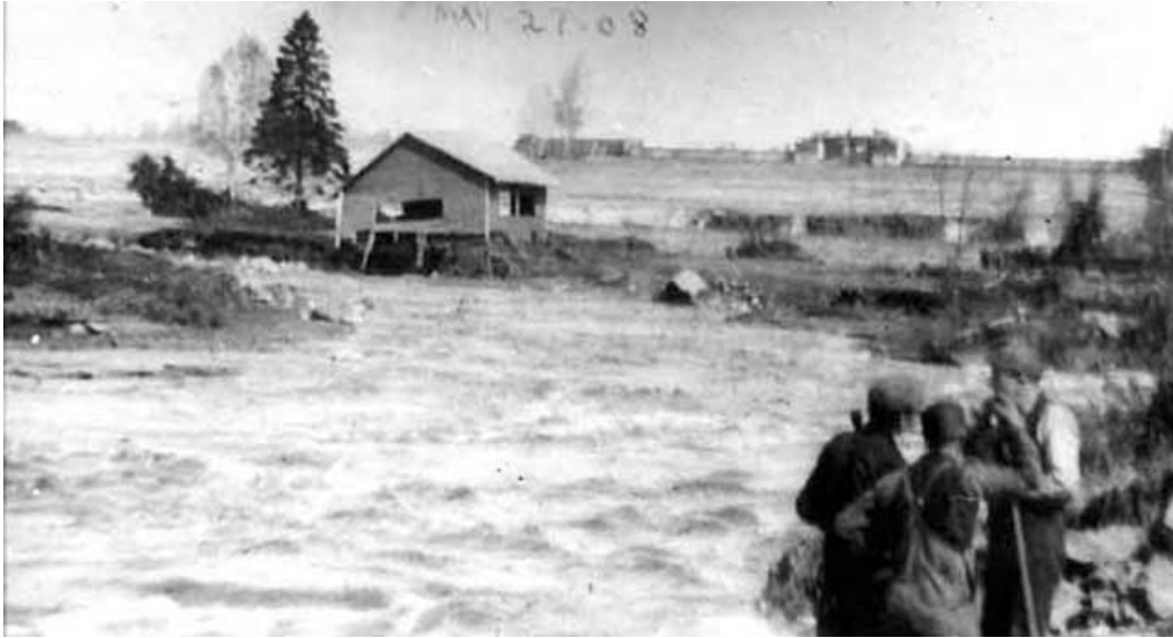
Looking upstream during the flood, 1908
