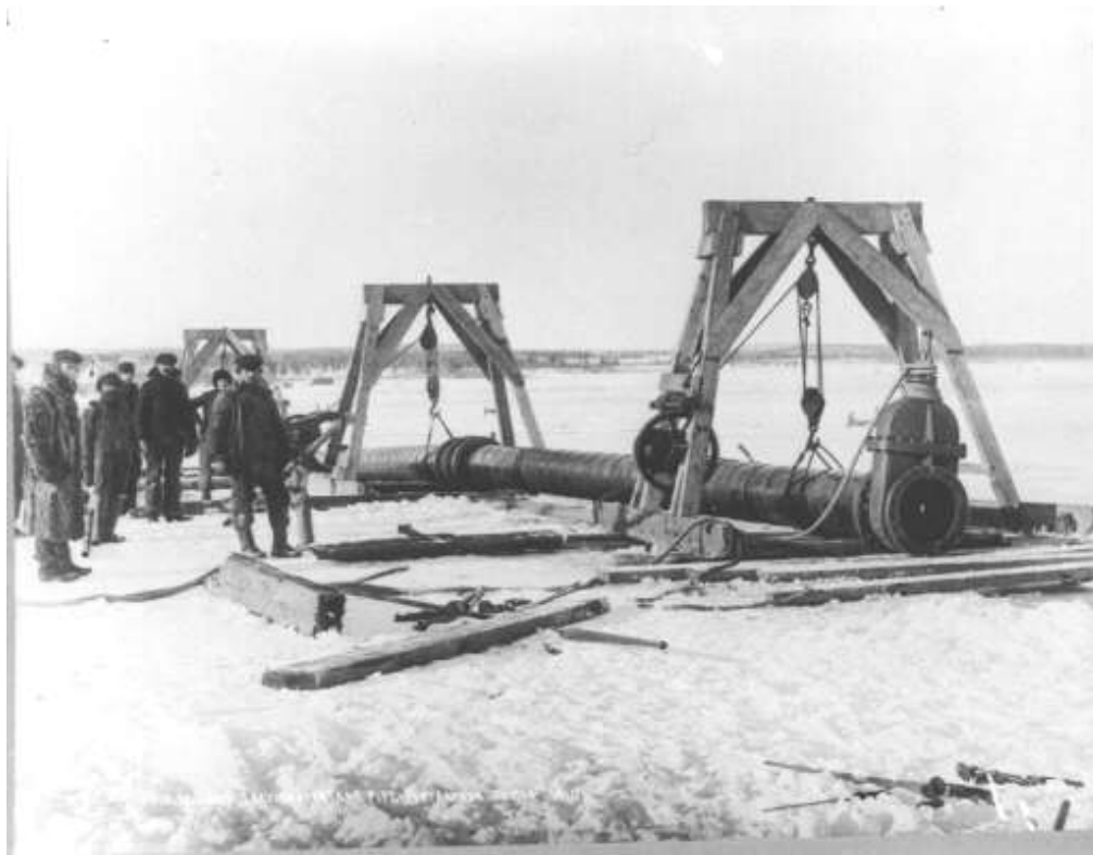
Installing the new water intake pipe off Bare Point, February 14, 1910.
