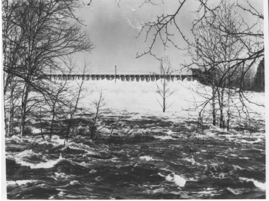
Boulevard Lake Dam, May 3, 1951.
