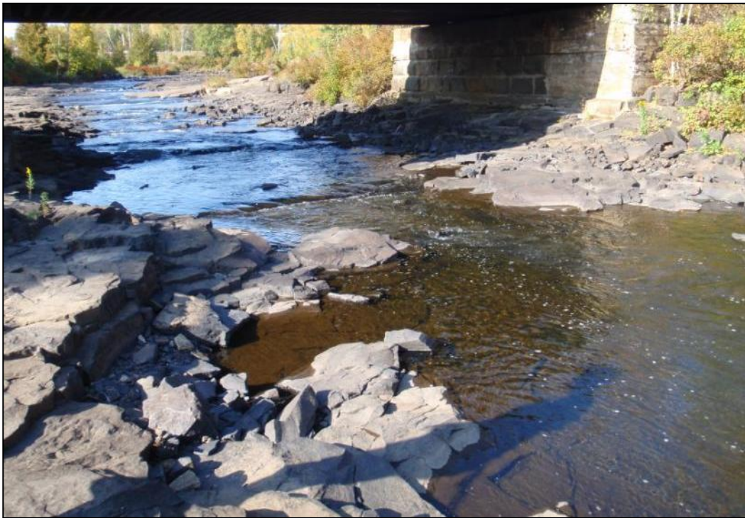
Reach #5 below 2 nd railway bridge looking upstream, Sept 27.
