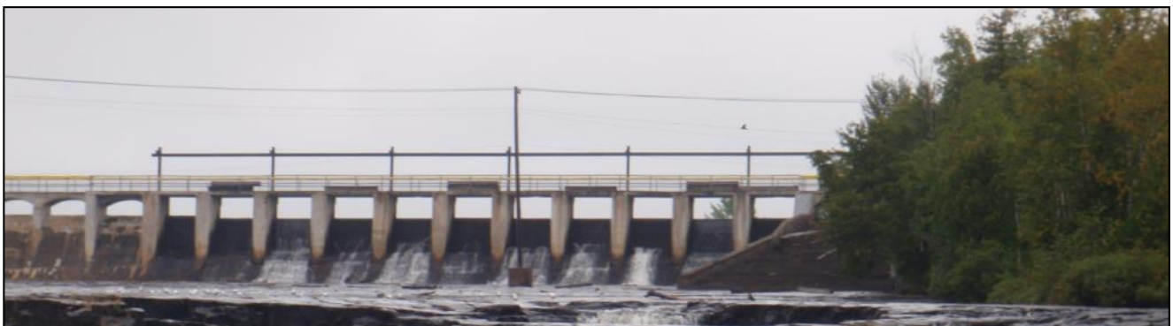
Figure 7. Leakage flows through the Boulevard Lake dam on August 31, 2011 during electrofishing.
