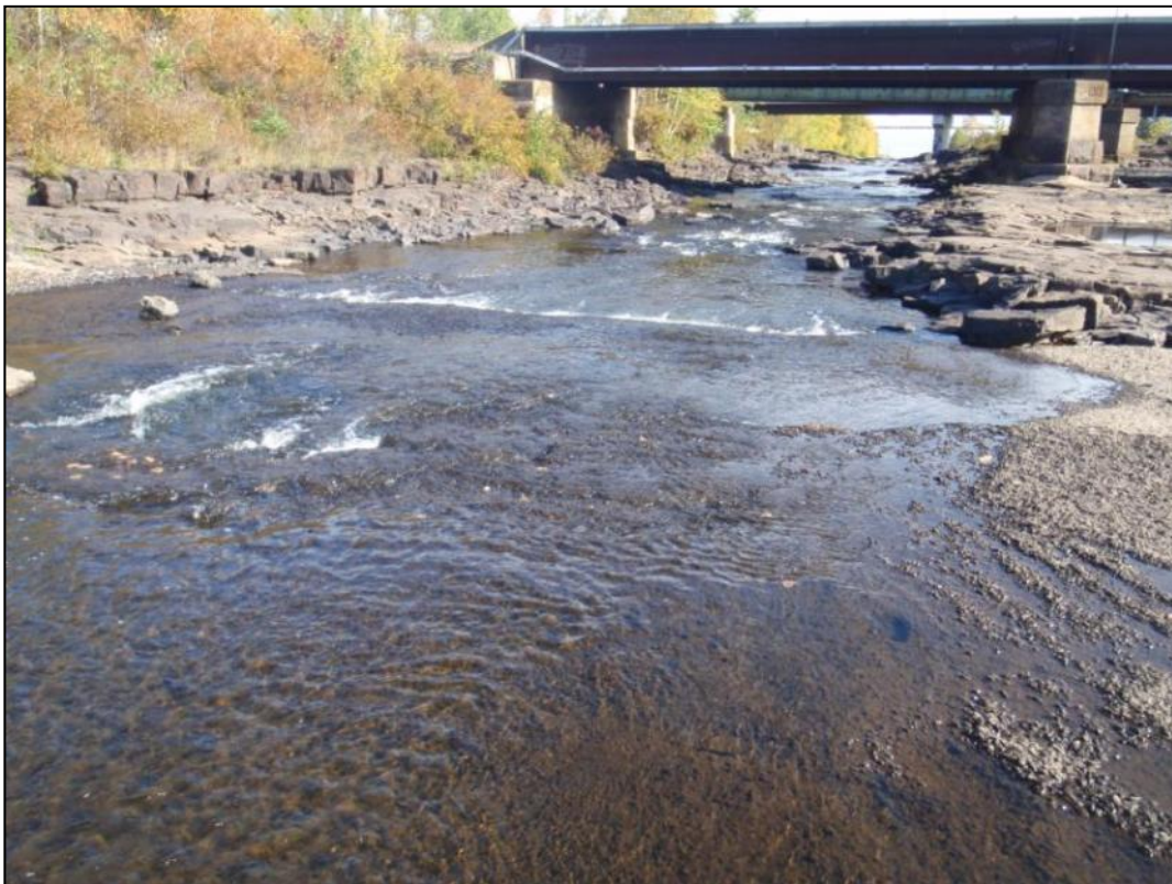
Concrete sheet in Reach #6 above 2 nd railway bridge looking downstream, Sept 27.
