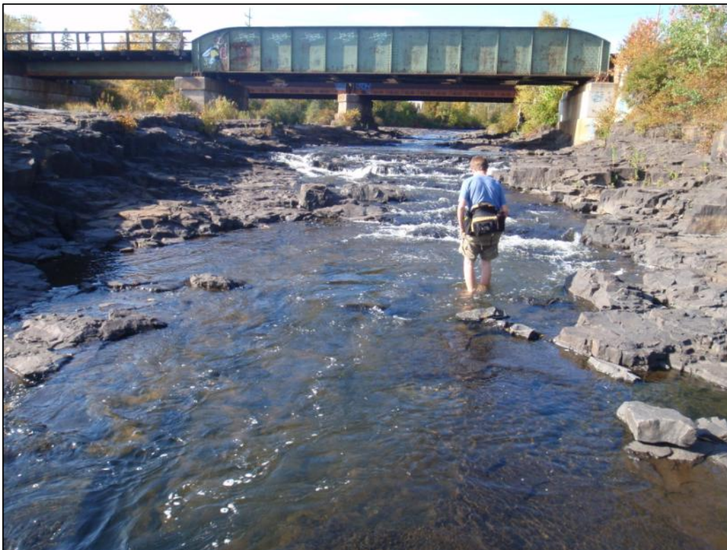
Reach #4 between Shipyard Road and first (downstream) railway bridge, Sept 27.
