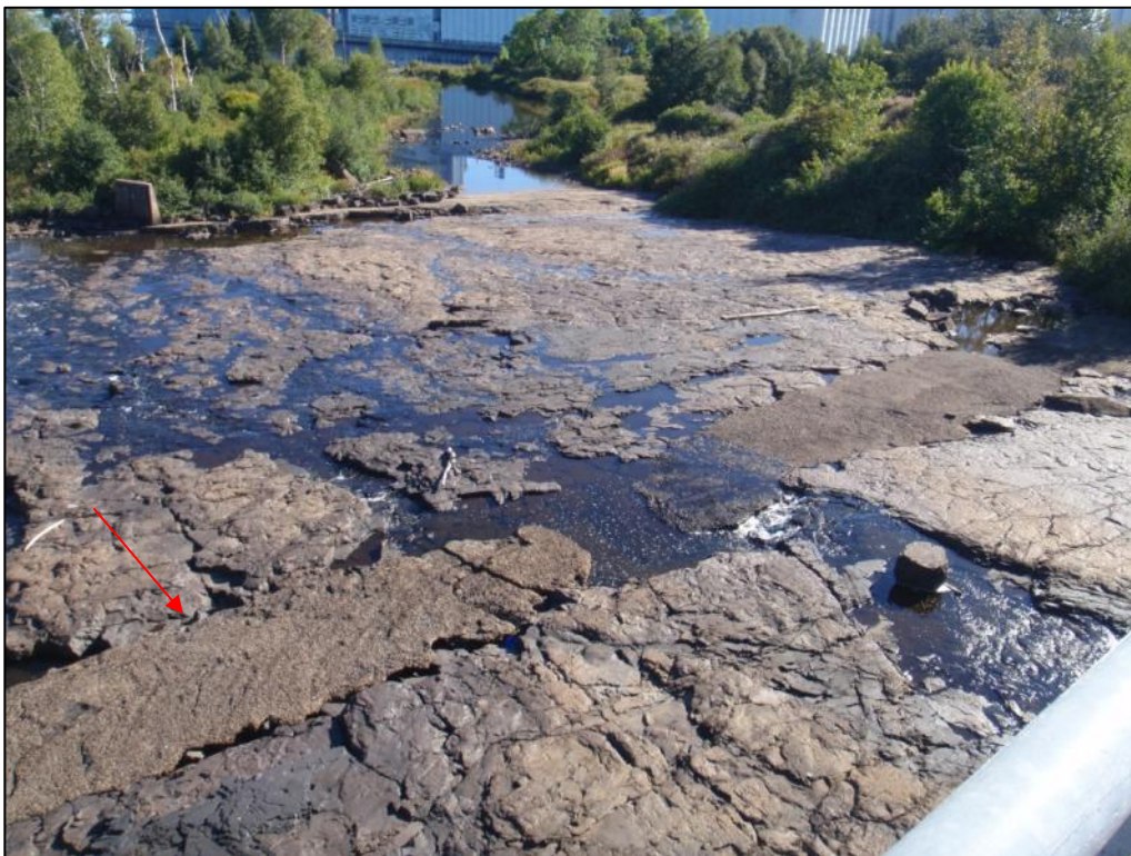
Figure 11. Current River below Shipyard Road, Sept. 9 looking at main (upper photo) and secondary channels (lower photo). Arrow denote band of concrete that cuts across channel.
