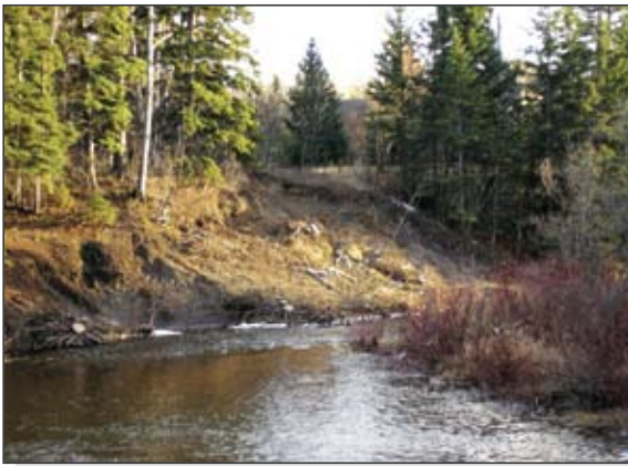
McIntyre River bank stabilization below Central Street bridge
